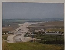
A505 Baldock Bypass constructed in 2003 using a cut and fill tunneling system.
