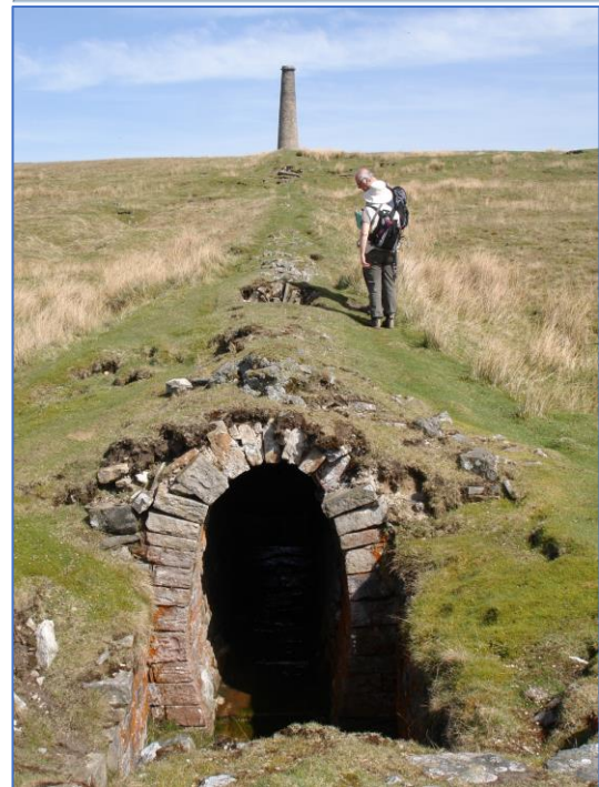
Condensate recovery flues from smelters Grassington, Yorkshire Dales (left) and Charterhouse, Mendips (right).
