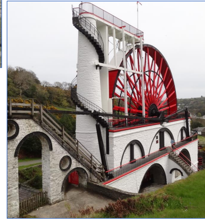
Laxey Wheel, Isle of Man, powers the mine pumps.
