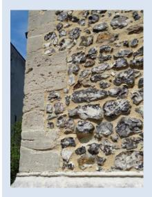
Fig. 2. The quoins of the tower buttresses are of limestone known as **Kentish Ragstone** (Cretaceous age) from the Maidstone area. Some have been replaced by **Bath Stone**.
