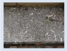
Fig. 14. War Memorial granite plinth showing large feldspar crystals
