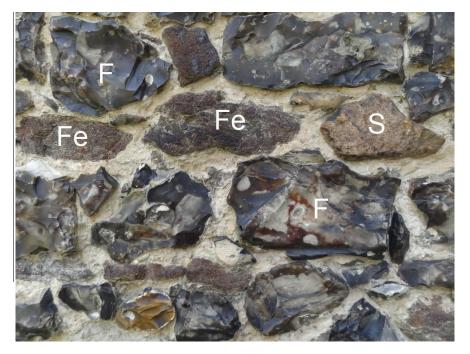
Fig. 1. Church wall showing flint (F), ferricrete (Fe) and sarsen (S)
